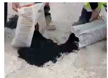
If the pothole is very deep, it is recommended, to apply the product in layers of 5 centimetres at a time to improve compaction with a bigger granulometry at the base (AC-25) and smaller above it (AC-11).
